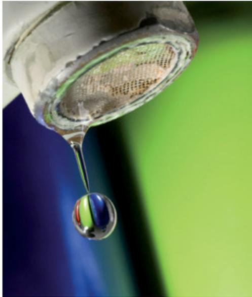
**Figure 11** Build-up of limescale on an aerating tap outlet.
